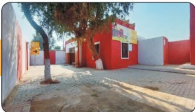
Repair & Renovation of BHU Gajan, District Jhal Magsi
