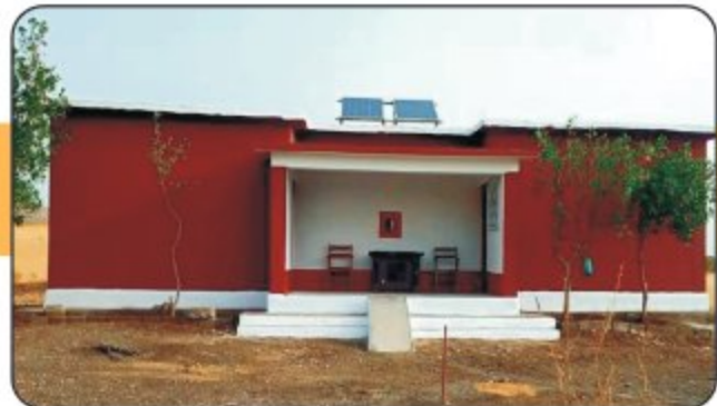
Repair & Renovation of BHU Koraro, District Khuzdar
