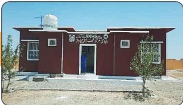
Repair & Renovation of BHU Pandandaz, District Panjgur
