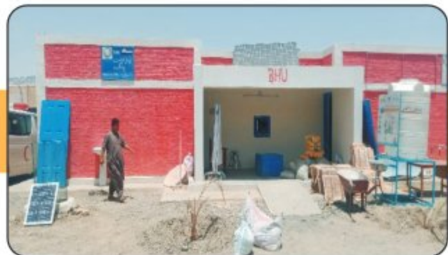
Repair & Renovation of BHU Padag, District Chaghi
